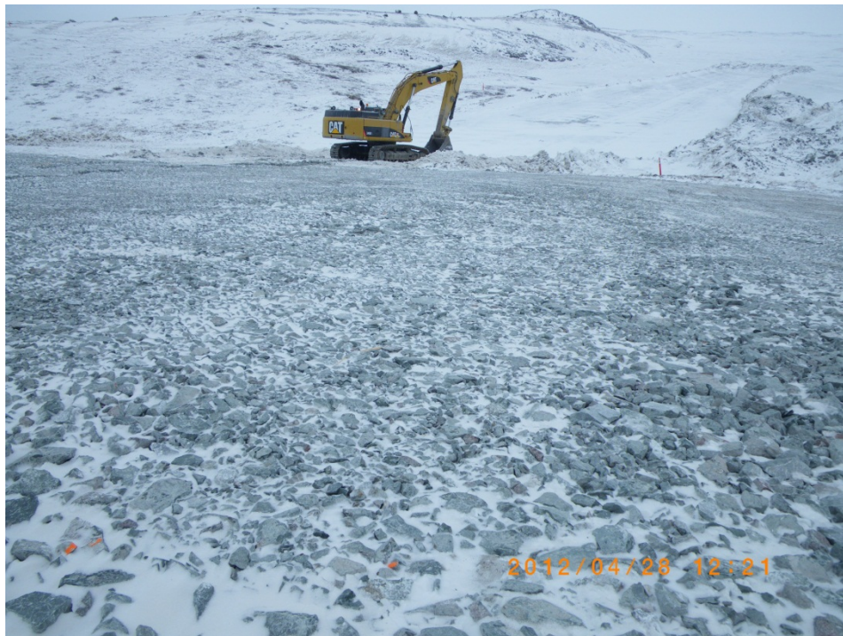
Photo 1: The final surface of the upstream face of the North Dam.
